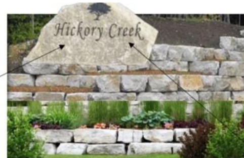
Built up Armor Stone Wall - higher on one side and signage on the other
